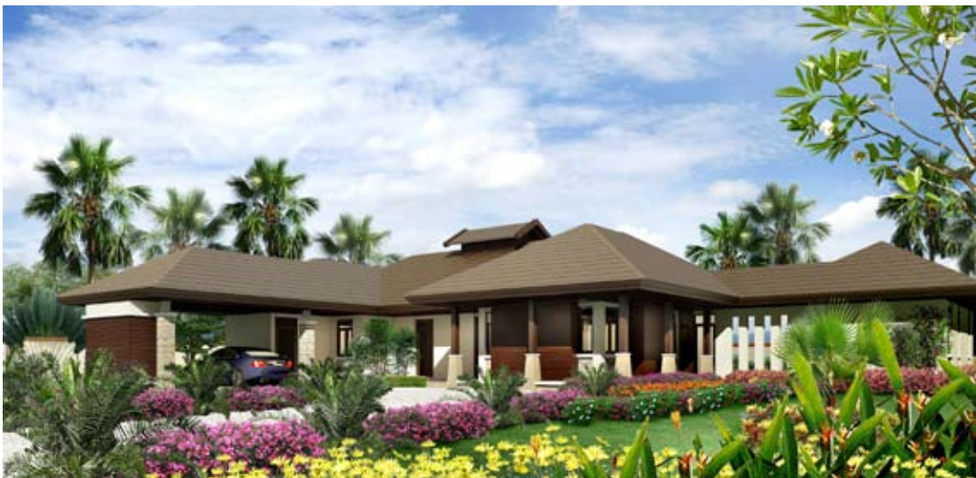
Image Above: What about this for a beautiful family home, country residence or super retirement house? Kensington is offering this luxury home with swimming pool, including 1 rai of land for 14.5 million baht. Check it out on www.thailandbuilders.com for further details.
